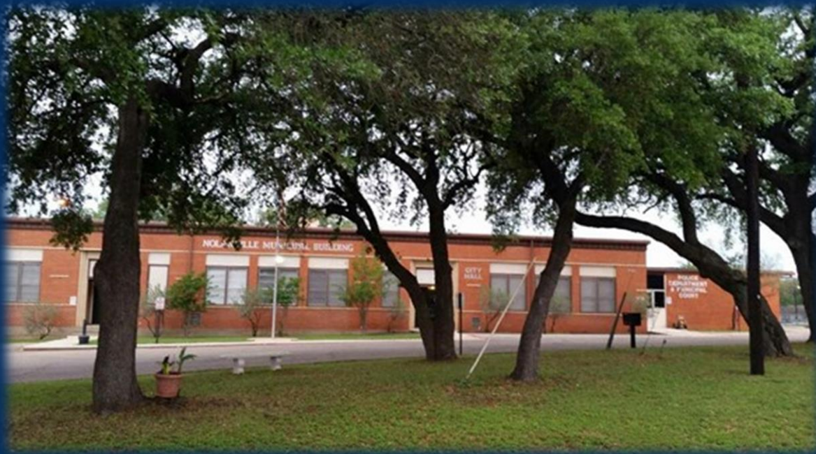
NOLANVILLE MUNICIPAL BUILDING 101 NORTH 5TH STREET, NOLANVILLE, TEXAS 76559
